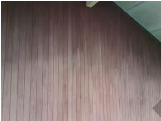
Typical Wood Veneer Fading
