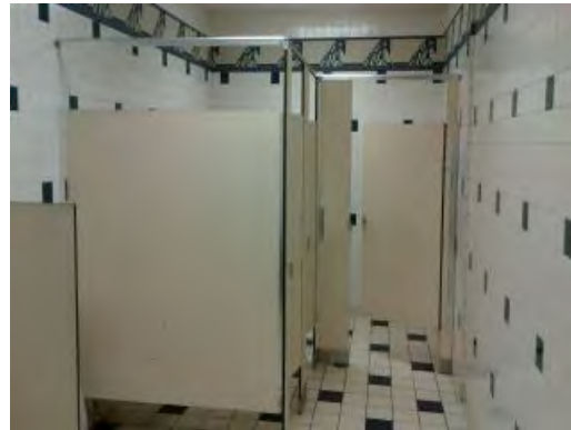
Boys 2002 Addition Restroom
