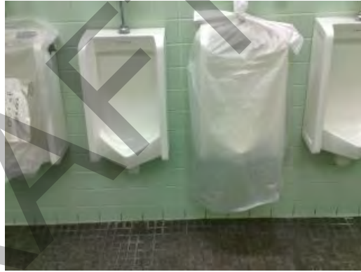
Main Building - Urinals Out Of Service
