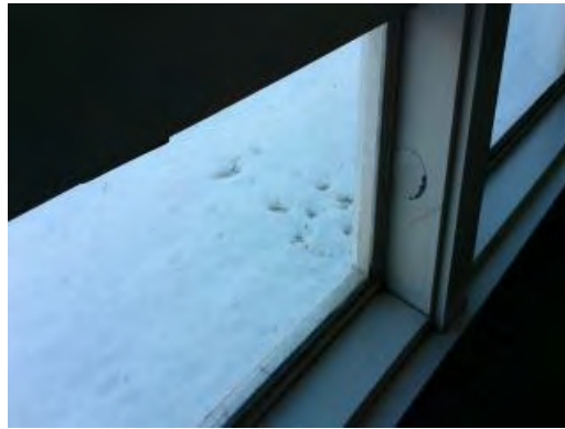
Main Building - Typical Single-Pane Window
