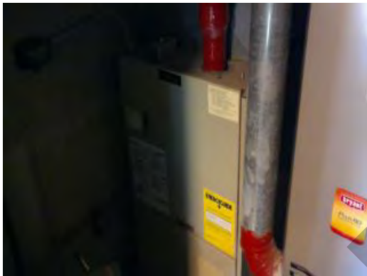
Corroding Furnace
