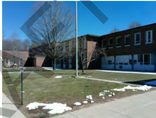
Main Building - Exterior
