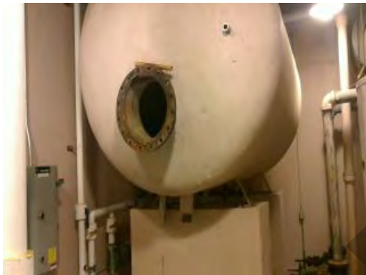
Main Building - Abandoned Storage Tank
