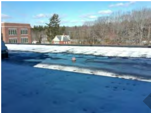
Main Building - Roof General Condition
