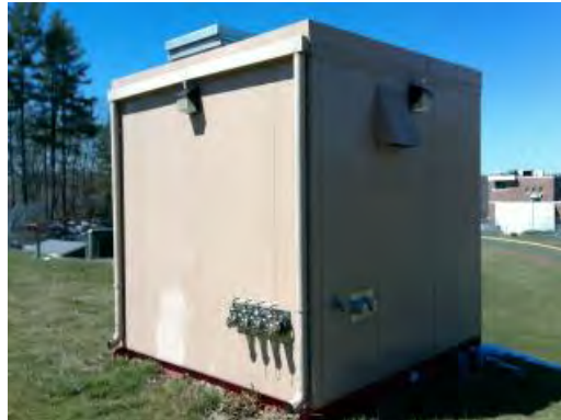
Fire Pump House - Exterior
