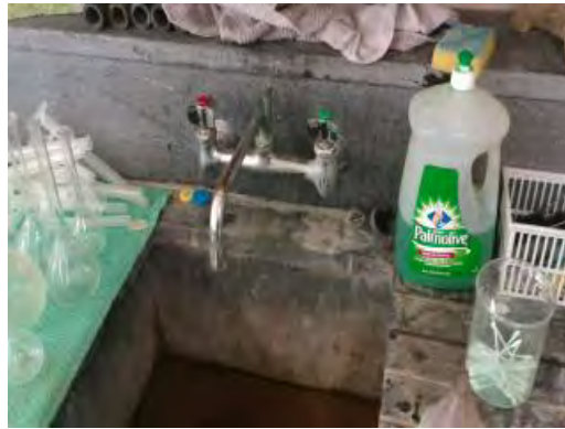
Main Building - Corroded Classroom Sink
