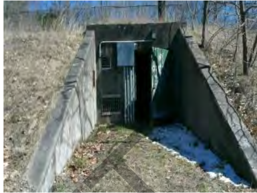
Pump House - Exterior
