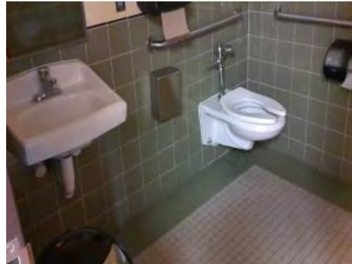
Restroom Fixtures And Finishes
