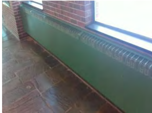
Main Building - Original Radiator
