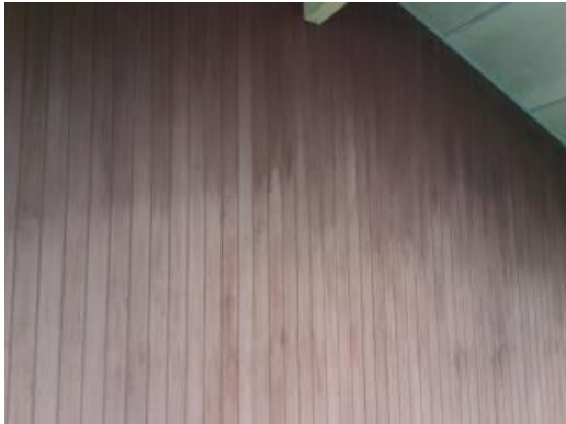
Typical Wood Veneer Fading
