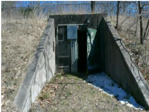
Pump House - Exterior
