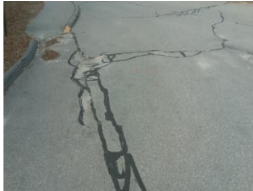
Damaged Asphalt
