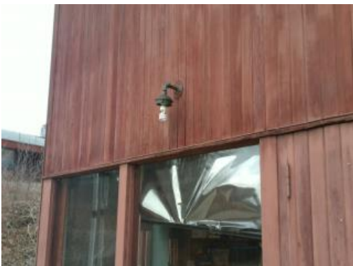
Building Mounted Light
