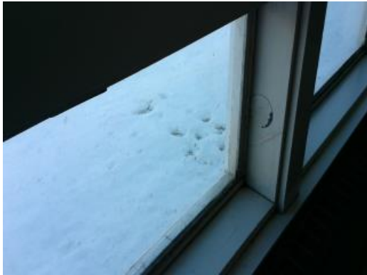
Main Building - Typical Single-Pane Window
