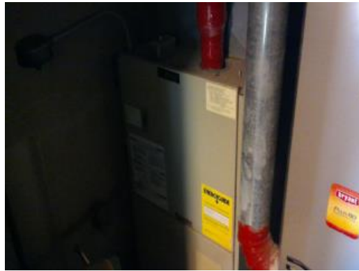
Corroding Furnace
