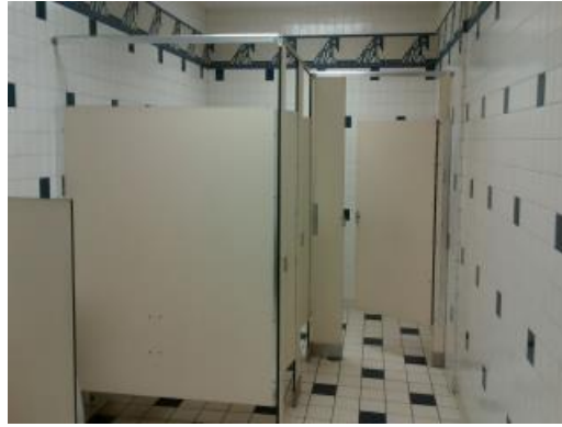
Boys 2002 Addition Restroom
