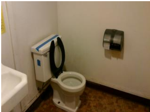
Typical Student Restroom
