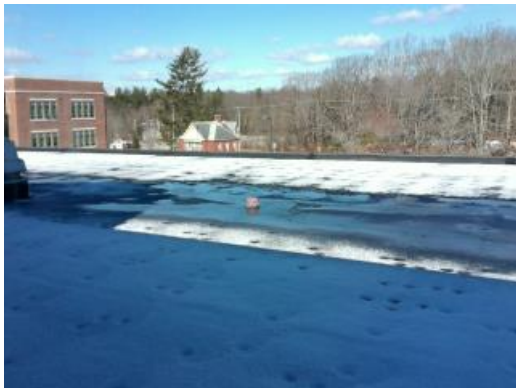
Main Building - Roof General Condition
