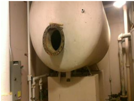
Main Building - Abandoned Storage Tank
