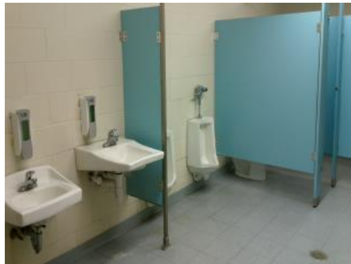
Typical Boys Restroom - 1989 Building
