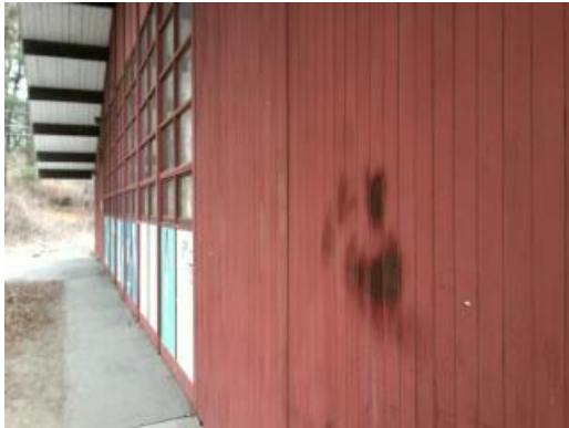
Stained Wood Exterior
