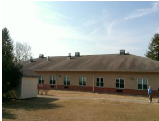
Original Shingle Roof
