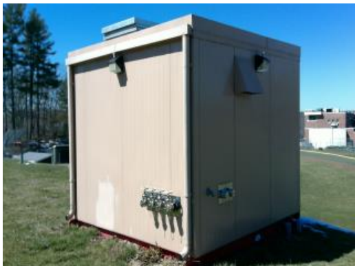
Fire Pump House - Exterior
