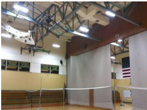
Main Building - Gymnasium
