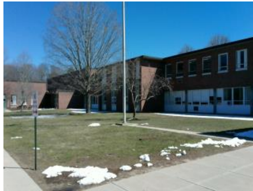
Main Building - Exterior
