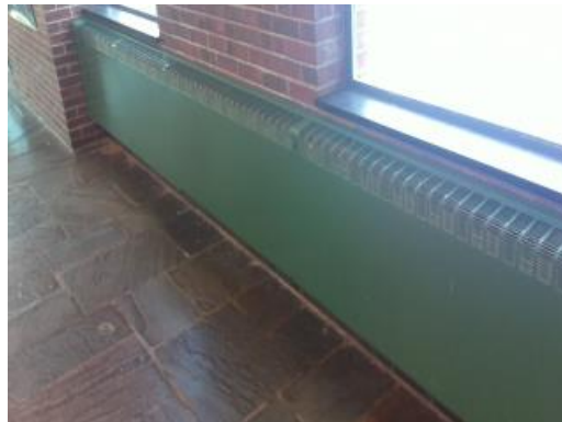
Main Building - Original Radiator
